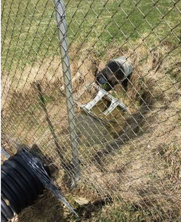
Storage Tank Overflow
