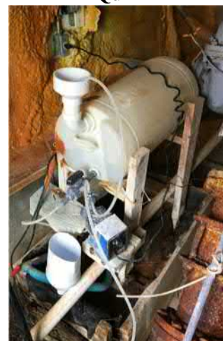
Chlorine Set-Up Well No. 2
