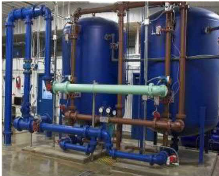
Ion Exchange Water Softening System
