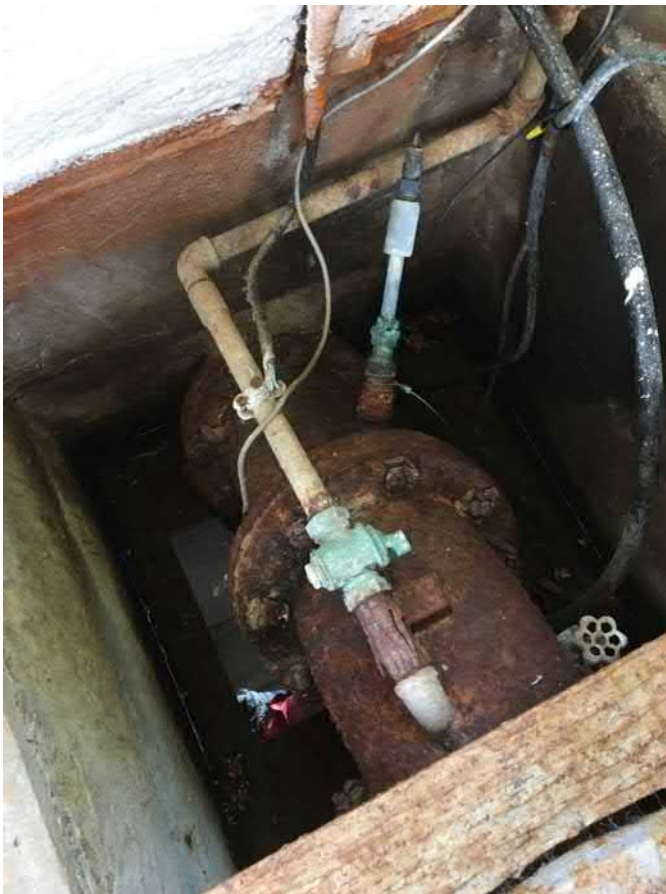
Well House No.1 Chlorine Injection Corp
