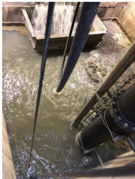
Before-and-after images show the effect of the PHi-CA large-bubble mixing system on a problematic lift station in Warwick, Rhode Island (C3ND Environmental Consulting).
