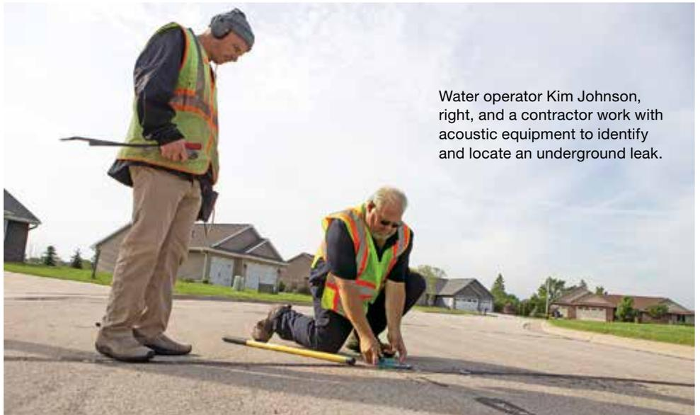
Water operator Kim Johnson, right, and a contractor work with acoustic equipment to identify and locate an underground leak.
